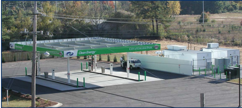
City of College Park, Atlanta Hartsfield Airport
